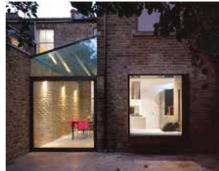
Best practice photograph An angled glazing providing daylight to the extension without overshadowing the neighbor
