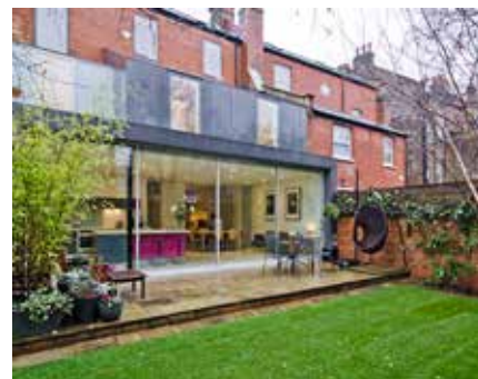
Best practice photograph A contemporary rear extension following the historical extension pattern
